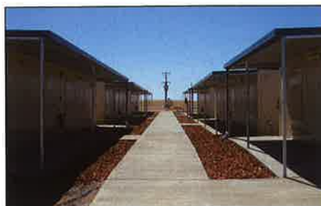
Example of the type of building to be supplied to Peculiar Knob.
